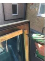
Remove any loose debris from the upstand and apply a generous bead of sealant to eliminate any draughts.
