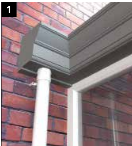
1 Return Cornice and guttering along host wall.
