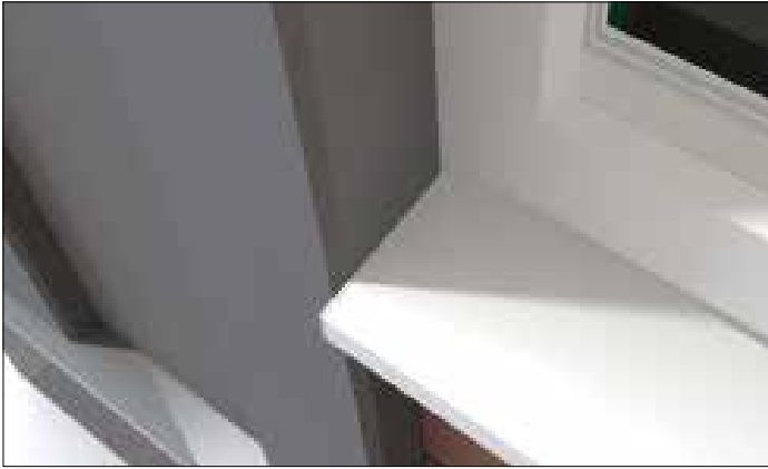
150mm PVCu cill against large column. Endcaps are required as cill will overhang the column claddings
