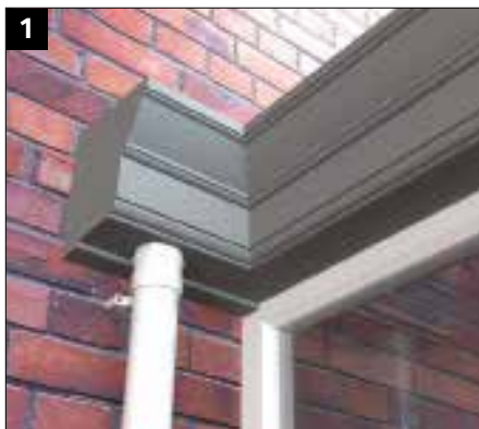
1 Return Cornice and guttering along house wall.
