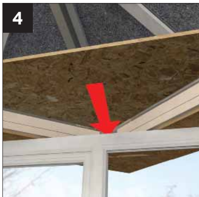
4 Slide into position additional external OSB board.
