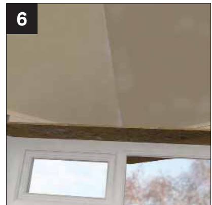
6 Plasterboard the roof.
