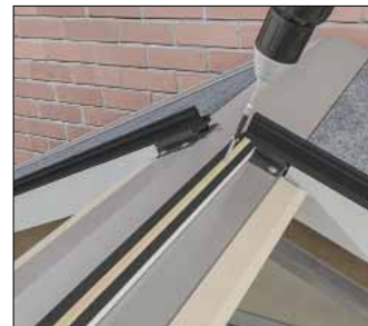
Fitting of the upper ridge glazing support trim
