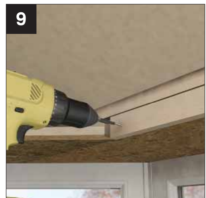
9 Attach additional mating timber battens.
