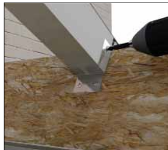
Fixing glazing bar at box beam shoe
