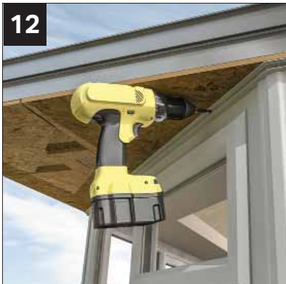
12 Fit external soffit channeling.
