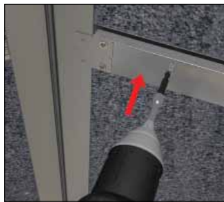
WPDS 020 3.5 x 50 Dry wall pozi countersink screw
