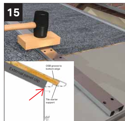
When aligned (ensure external panel clip butts upto aluminium gutter channel, see red arrow) use a robust mallet to knock down the external panel locking clips (use a short length of timber to protect the clip from indentations).
