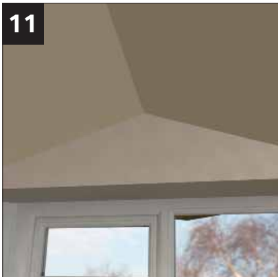
11 Plasterboard face of gable
