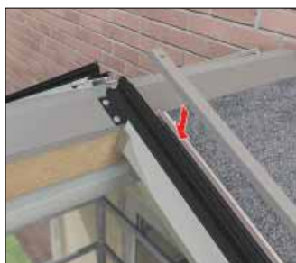
Fixing glazing bar to ridge
