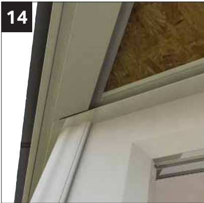
14 External ship lap cladding edge channel detail.
