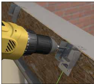
Fixing glazing bar shoes at box beam
