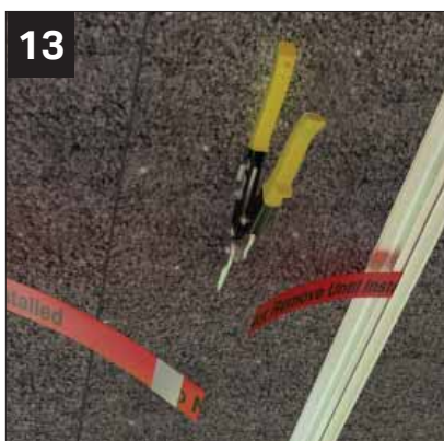
With the expandable panel in position, snip all the retaining straps.
