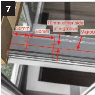
The 4 fixing positions.
