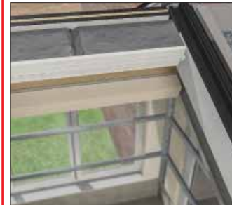
Fitting upper plasterboard trim
