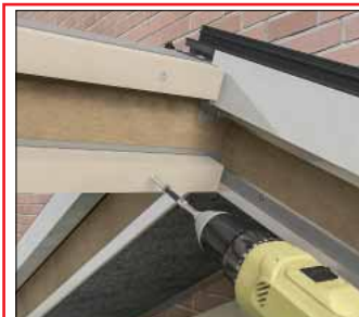
Fitting of the timber ridge battens
