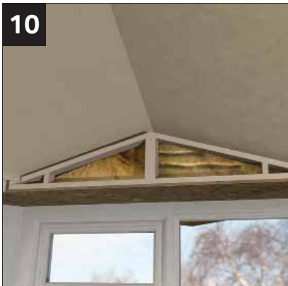
10 Insulate void with mineral wool.
