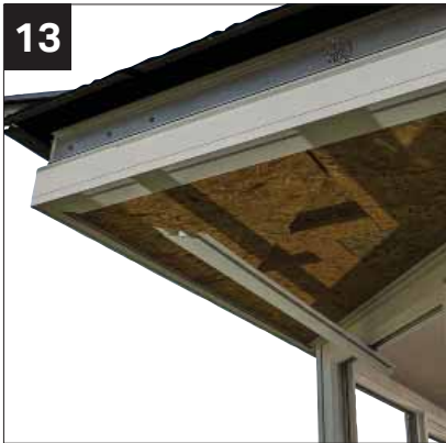
13 Fit external ship lap cladding edge channel.
