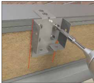
Fixing glazing bar shoes to ridge section
