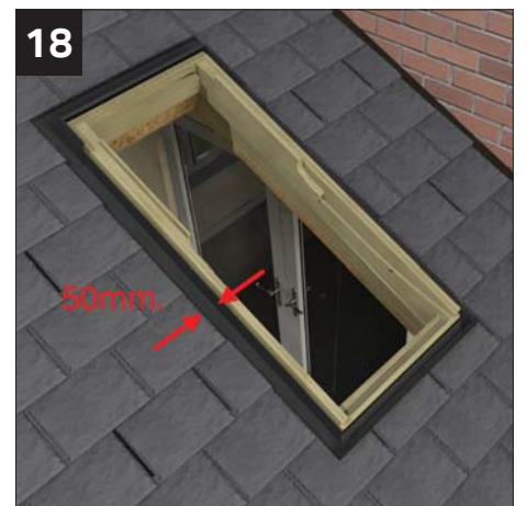
18 Fit the tiles following the relevant information shown on pages 28 to 33. The tiles should be centred around the Velux with a 50mm gap to the left and right sides.
