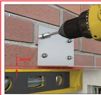
Fixing hanger bracket to wall
