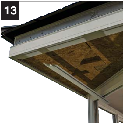
13 Fit external ship lap cladding edge channel.
