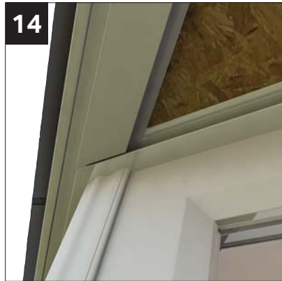
14 External ship lap cladding edge channel detail.
