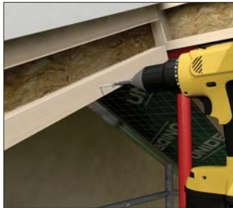
Re-fitting panel timbers
