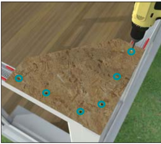
Fixing support shelf to existing frames
