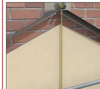
Fixing ridge hanger to the wall
