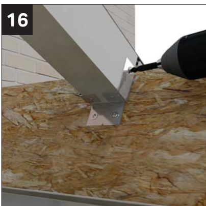
16 Fix all glazing bars into box beam shoes, again, using 4 x (NRTS 050) for shoe (NRBE001) or 6 x (NRTS 050) for shoe (NRBE002) provided.
