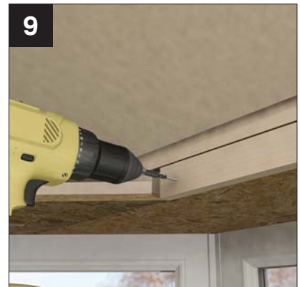
9 Attach additional mating timber battens.
