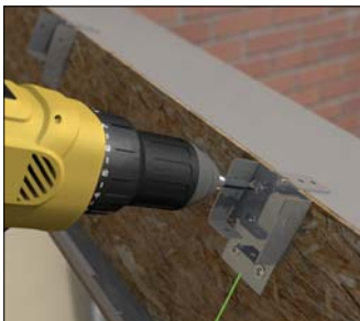
Fixing glazing bar shoes at box beam
