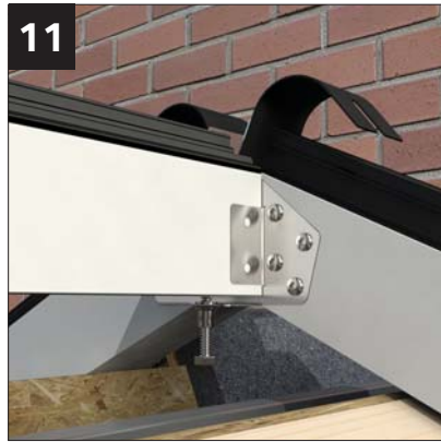
11 Adjust glazing ridge beam height using thumb screws to ensure glazing gaskets are in aligned.
