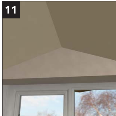
11 Plasterboard face of gable
