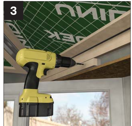
3 Attach additional battens.
