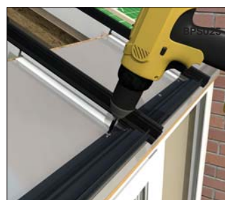
Fixing glazing support section
