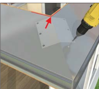
Securing upper box beam cleats
