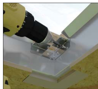
Fixing hip bar support brackets
