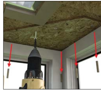
Fixing beam to corner
