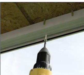
Fixing through head of window frame into beam
