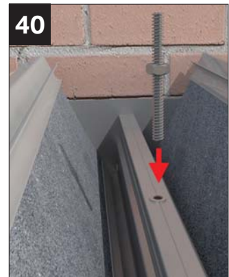
Assemble nut and threaded bar. Screw down into ridge body. See note below.
