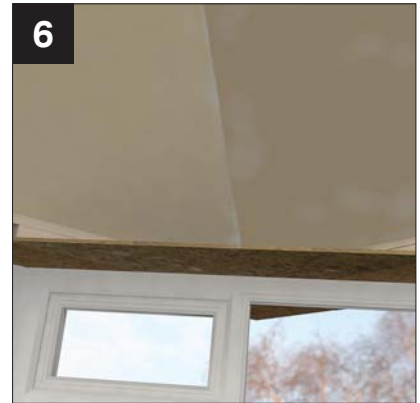
6 Plasterboard the roof.
