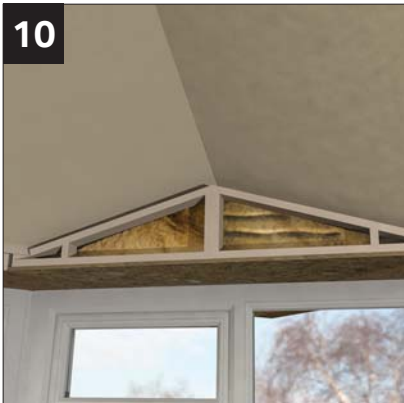
10 Insulate void with mineral wool.
