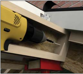
Fixing through purlin into cassette
