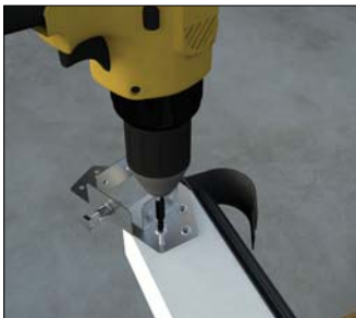
Fixing glazing bar adjustable connection bracket
