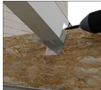
Fixing glazing bar at box beam shoe
