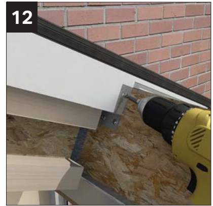
12 'A' frame being fastened into box beam shoe.
