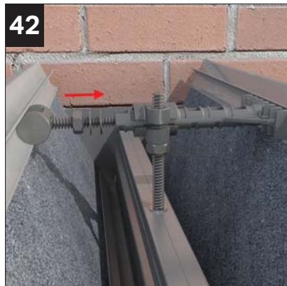
Ensure coupler assembly is finger tight into panel extrusions.
