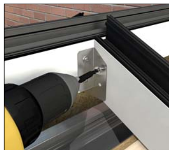
Fixing glazing ridge to glazing bars
