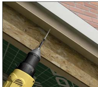
Securing glazing bar against panel timber
