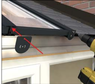
Fixing glazing bar end caps
