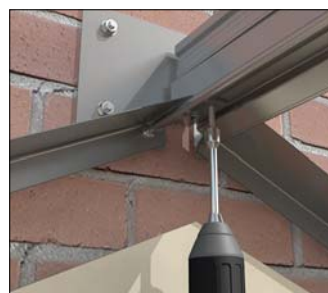
Fixing ridge to ridge hanger
