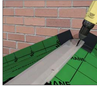
Fixing ridge under capping into tile stop
