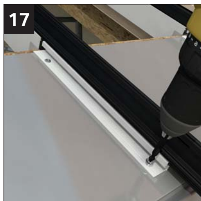
17 Secure glazing bar to external face of box beam. Two screws each side using (NRTS 050) provided.
