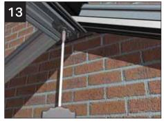
Ensure that the fixing on the eaves moulding and the nuts on the 'crocodile hanger' are tightened up.
