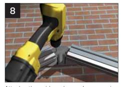
Attach the ridge hanger/compression plate to the host wall. Drill the plate with 2 x 9mm holes, then the wall with an 8mm masonry bit and fasten into the masonry using the two M6 x 65mm sleeve anchors (or resin anchors) provided. If necessary, use aluminium shims to pack out behind the plate. Check the plate is vertical and securely fastened. AT THIS STAGE IT IS ADVISABLE TO CHASE OUT FOR CONSERVAFLASH/LEAD FLASHING.
