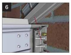
Attach the starter bar using the nut, bolt and spring washer (included in the kit) to the eaves structural moulding. Finger tighten the nut to temporarily allow the assembly to hang.
