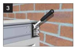
Where the eaves beam sits against the host masonry wall, it has a structural moulding attached to the eaves beam. This has three fixing positions cast into it to allow attachment into masonry – choose the hole that directly lines up with solid masonry and drill a 10mm hole into the host wall. Attach the structural moulding using the M8x80mm anchor supplied. Silicone seal the gap where the moulding attaches to the eaves beam.
