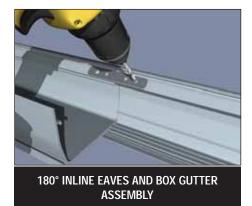
Place the inline cleat (SES002) over the butt joint. Fix down either side of the joint with the two fixings supplied (UZBGF001-D).
