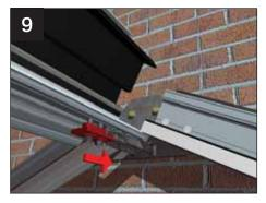
Loosen the "crocodile jaw" bolts on the underside of the main ridge body – ensure it is supported at the front whilst it is gently guided onto the top half of the 'crocodile jaw'.
