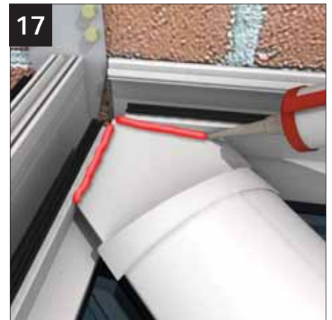
Silicone valley topcap against ridge wings
