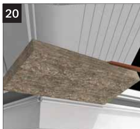
Cut two 200mm lengths of valley undercladding. These will act as templates for top and bottom scribes. Use a 'straight edge' placed tight to the eaves fascia board, then mark and cut.
