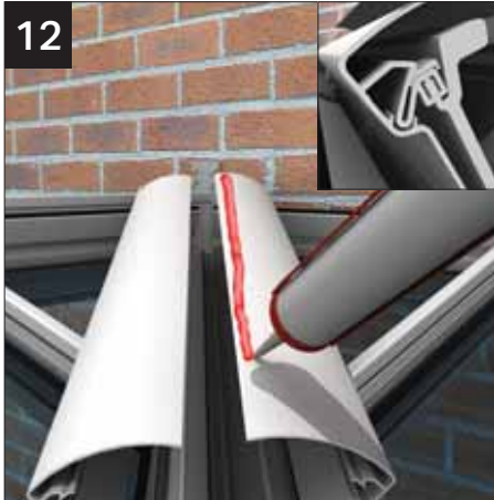
Fit one half of the valley cladding ensuring that clip locates over aluminium barb. Silicone down the length of fitted cladding
