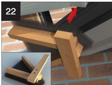
Offer up the cassette assembly into position.
