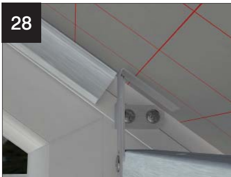
28 where panel adjacent to the gable is solid - the channel spans from insulated internal pelmet frame up to ridge detail and should be fitted directly below the 90mm insulation (insulated internal pelmet detail shown).
