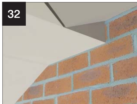
Now fit the plasterboard – the detail where the valley abuts the host wall should look as shown. Fitters tip: fit the small triangular segment of plasterboard shown first, allowing space for the upper adjacent board to slide in above it, as there will be nothing to screw to at this point.
