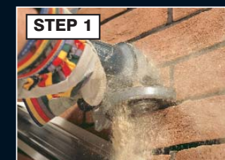
Chase out with grinding wheel
