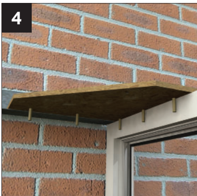
4 Lower into position: Tight back to angled wall bracket. Position dowel guides tight to internal frame
