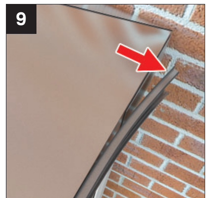
9 Lever the aluminium gutter support channel outwards to enable the external beam cleat to slide behind.
