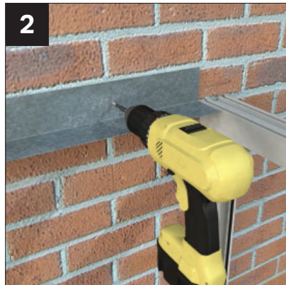
2 Place centrally, aligning top face with head of frames. Bolt to host wall using masonry anchors suitable for substrate (avoiding mortar joints)
