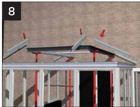
8 Now the Pagoda eaves beam is assembled into a one piece structure, temporarily support it. Attach the glazing bars according to the component location plan. Tighten the bars, at the pagoda beam end first and then at the main eaves beam second.
