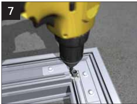
7 If supplied, fasten to each corner the tie bar drop rod fixing bracket to the underside of the pagoda eaves beam.
