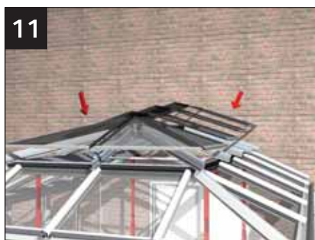
11 Glaze the upper pagoda roof, and complete all external works
