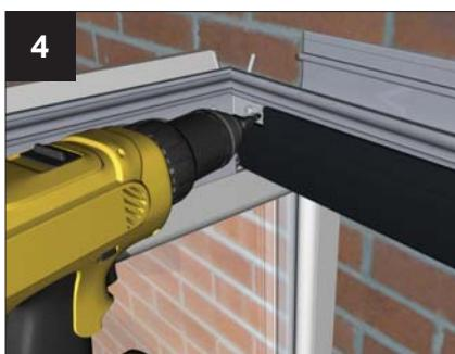
Either peel back or knife off a small amount of the insulation where the cleat is to be fixed. Drill a 4.5mm pilot hole and then fix the cleats with the two M5 12mm tap-tite screws provided. The protruding tap-tite screws will need trimming back prior to fixing the adaptor (alternatively, when its time to insert the adaptor, undo the tap-tites, drill a pilot hole through the adaptor and then re-screw the tap-tites and fully seal).
