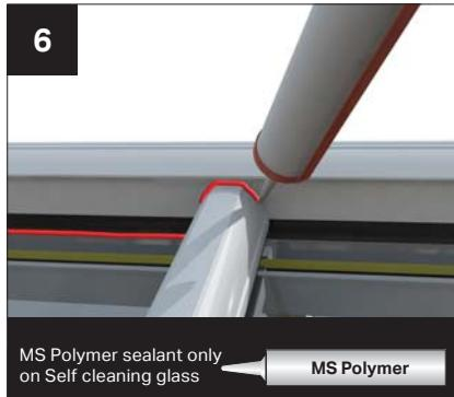
Seal along the ridge baffle where it meets the glazing and over any bar where it meets the ridge.
