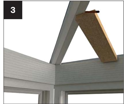
3 Use the location plan again for the hip positions. There will be a left and right. Mark these positions and then line up bracket and attach as before.
