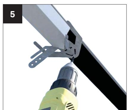
Take the corner bracket CHA090 and attach using 4.2x19mm self drill pan head screws (supplied). The back edge of the bracket should butt up to the under claddings.
