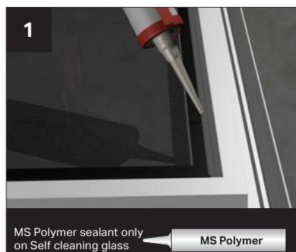
Seal the area around the full perimeter of the glazing.
