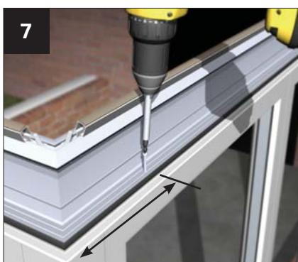
Securely fit the eaves beam to the frames using for example, 38mm x 4.8mm screws in the position shown. Fix down at 450 centres and within 200mm of each corner.
