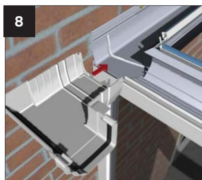
Slide the adaptor into the aluminium box gutter, raising up its front edge to utilise the unique 'snow plough' effect. This spreads the Gutterbond evenly under the adaptor. Push the adaptor firmly up to its end stop, so that it will line through with the Classic gutter attached to the eaves beam.
