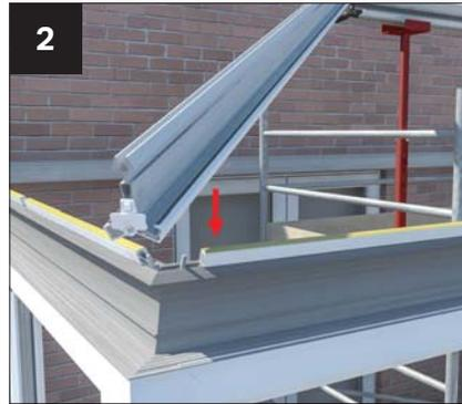
2 If not already attached, attach the glazing bar end cap fixing blocks - as access restrictions may prevent easy fixing later. NOTE: These 'snap out' of the end caps when dispatched from the factory. remove nuts on eaves beam. Fit hip bars onto bolt sat eaves end and hand tighten nuts.
