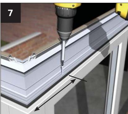
Securely fit the eaves beam to the frames using for example, 38mm x 4.8mm screws in the position shown. Fix down at 450 centres and within 200mm of each corner. For 60mm frames use the inner eaves extrusion line and outer line for 70mm frames. Always screw down. (Not supplied)
