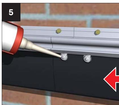
Now seal over all the exposed bolt heads, on the inside and outside of the box gutter.
