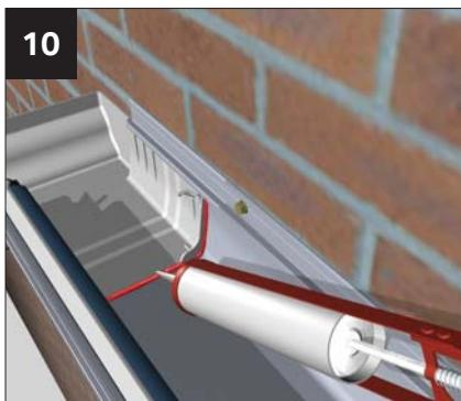
Use the balance of the Gutterbond to back point any gaps at the front edge.
