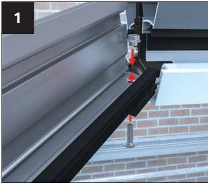
1 Offer up the top bars to the ridge and attach loosely using the roofing nuts and bolts supplied. SHBC001S
