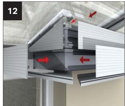
Internally, cloak off the open end of the glazing bar by fabricating a small end closure – seal into place. Fit the lower fascia and boxgutter claddings in the usual way. Scribe and secure the upper claddings to the factory applied horizontal sticky tape strips. (For raised back box gutters beyond 300mm in height, vertical claddings must be fabricated from your own supplied multi board).
