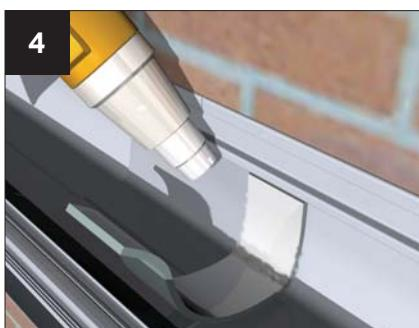
Check surfaces are dry, clean and grease free. De-grease if necessary.
