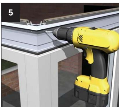
Using the pre-drilled pilot holes, drill two 4.5mm holes through the corner cleats.
