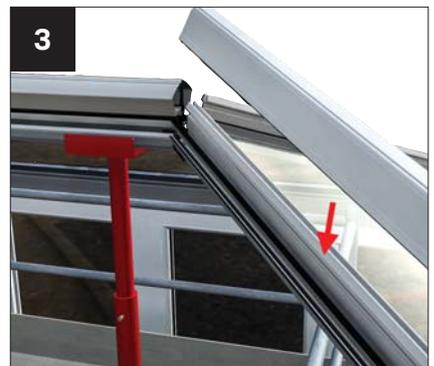
Work your way around the roof and fit glazing bar top caps.
