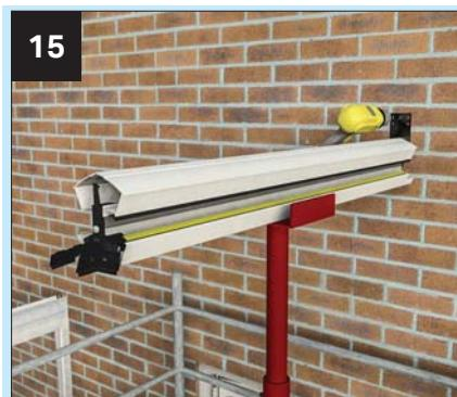
Using the roof rise height supplied set the ridge and fix the bracket to the host wall using the appropriate fixings.
