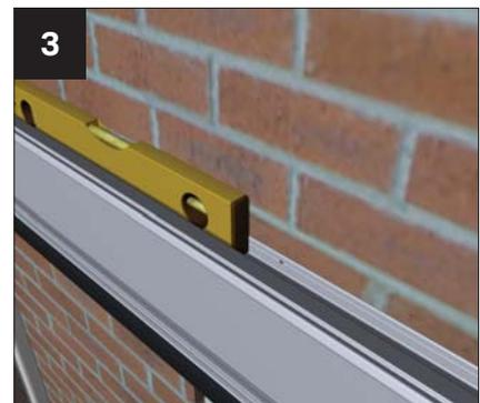
Lift the box gutter back into position, check levels, and then mark the wall (through the pre-drilled holes) ready to drill the host wall and grind out for the flashing.
