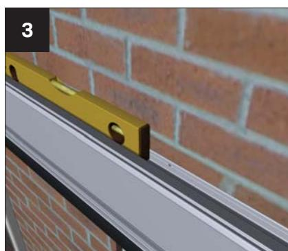
Offer the raised back or special box gutter into position. Carefully mark onto the aluminium leg against the host wall the position of each fixing – use 600mm maximum centres.
