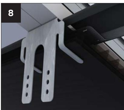
Push the polycarbonate up to the roof and bend the long legged tabs to hold the panel in its final position.
