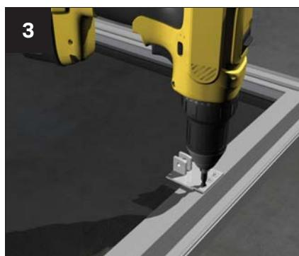
Centrally screw fix the sash bracket into the position shown above using the fixings provided. Leave the sash to cure before fitting.
