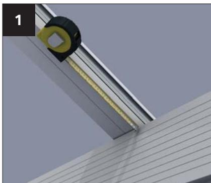
Using the location plan find the dimension for setting the bracket position. Measure up the bar from the top edge of the fascia board and mark.
