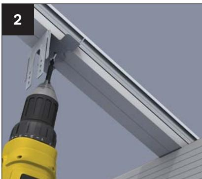
As above and ensure back edge of bracket butts up to pencil line.
