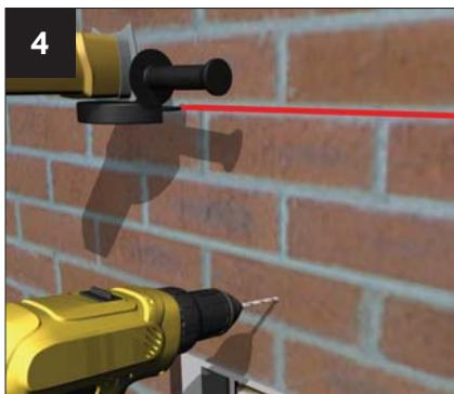
Remove the box gutter and drill the host wall where marked. Grind out the course which is at least one course higher than the raised back height.
