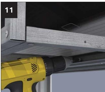
Check the frame is level and and fix either on or below fascia wing using 4.8 x 32 self-drill screws provided.
