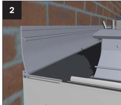
Place eaves beam section – with undergutter trim attached – onto the side frames. Seal the joint between the eaves beam and box gutter.
