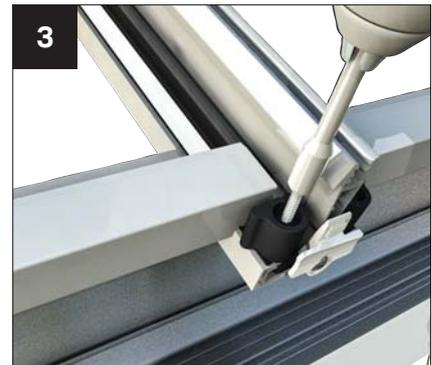
3 Centralise the glazing between the glazing bars. If necessary, pack out on each side. Now fully peel away protective film from glazing support at eaves and ridge and press glazing down firmly. Ensure that glazing end profile sits snugly behind grommet, on the glazing end stop. Now using the fixings provided, screw down into the bar as shown.
