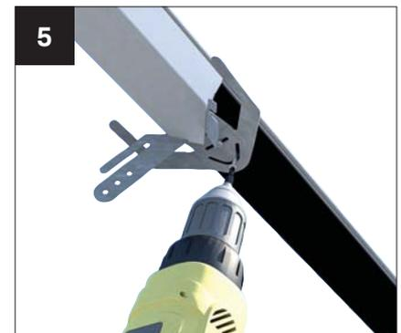
5 Take the corner bracket CHA090 and attach using 4.2x19mm self drill pan head screws (supplied). The back edge of the bracket should butt up to the under claddings.
