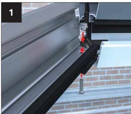
Offer up the top bars to the ridge and attach loosely using the roofing nuts and bolts supplied. SHBC001S
