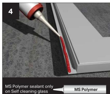
With the opening sash removed, lay the mainframe upside down on a smooth clean surface (protect the surface to prevent damage). Run a continuous bead of sealant (appropriate to the glass type) immediately behind the co-extruded gasket on the upper and lower legs.
