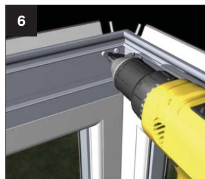
Securely fit the two M5 x 12mm taptite screws.
