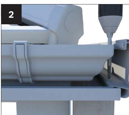
Offer up the middle Cornice section into position, (it may be advisable to temporarily support the lower Cornice section whilst fixing) secure using fixings provided (CRN007). (Long reach driver required).
