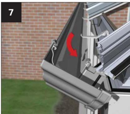
7 Locate the back edge of each section of gutter into the slot in the gutter bracket.
