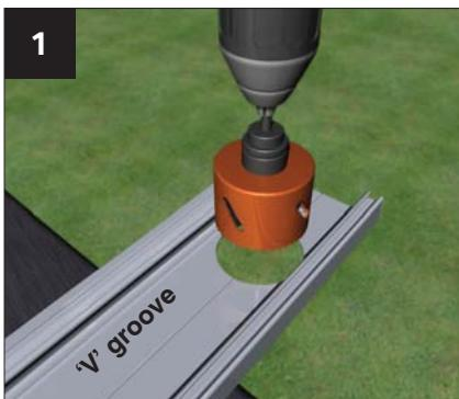
Decide the position of the gutter outlet by lining the extrusion 'v' groove up with the centre of the hole for the down pipe. Using a 73mm dia hole saw, cut the hole for the down pipe in the lower section.
