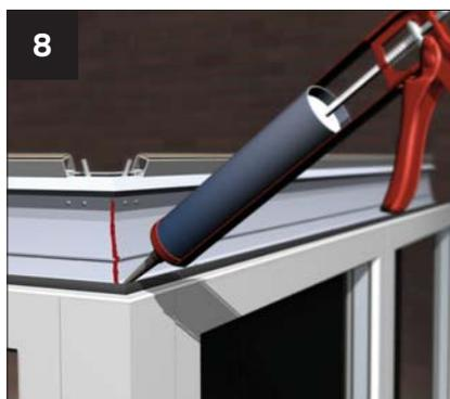
Once the eaves beam is secure, run a bead of silicone down the joint where the eaves beam sections meet and where the eaves abuts the host wall.
