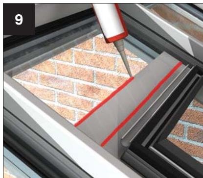
Using appropriate sealant (low modulus neutral cure for polycarbonate and MS Polymer for self cleaning glass), run beads along top and bottom edges of both H sections.
