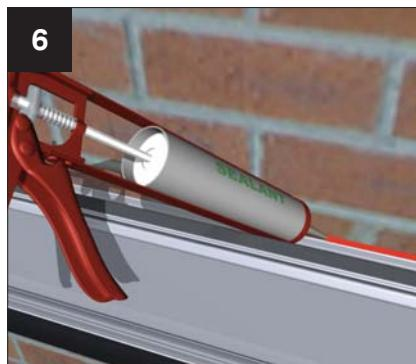
Seal the top and bottom edges of the box gutter and follow all other steps as per standard box gutters on page 21-22. When installing the lead flashing, ensure that the top of the flashing is higher than the point of rain water discharge from the glazing bars. Clad off the deep skirt of the raised back box gutter using multi-board (not supplied).
