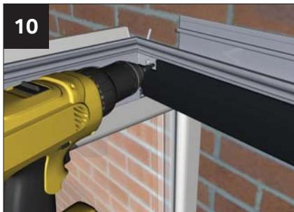
Either peel back or knife off a small amount of the insulation where the cleat is to be fixed. Drill a 4.5mm pilot hole and then fix the cleats with the two M5 12mm taptite screws provided.. The protruding taptite screws will need trimming back prior to fixing the adaptor (alternatively, when its time to insert the adaptor, undo the taptites, drill a pilot hole through the adaptor and then re-screw the taptites and fully seal).
