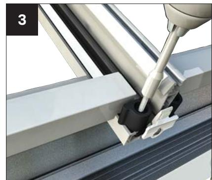
Centralise the glazing between the glazing bars. If necessary, pack out on each side. Now fully peel away protective film from glazing support at eaves and ridge and press glazing down firmly. Ensure that glazing end profile sits snugly behind grommet, on the glazing end stop. Now using the fixings provided, screw down into the bar as shown.
