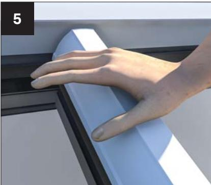
Using the heel of your hand, push down on the top cap to engage the clips, working from ridge to eaves. Ensure the rubber gaskets are full compressed for a watertight seal. NOTE: on longer bars it may be necessary to use a soft mallet and timber block
