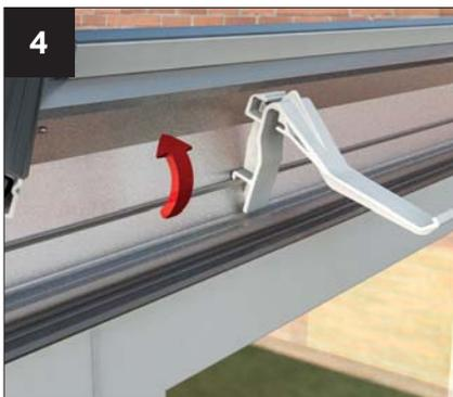
4 Fit all the gutter brackets supplied with the kit at maximum 750mm centres and maximum 200mm from each corner.
