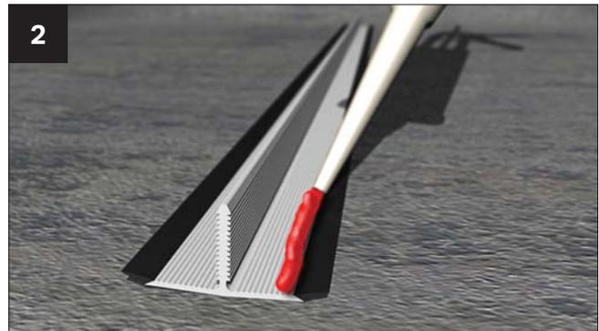
2 Now take the upper section and lay it face down onto a smooth clean surface. Using the relevant sealant (MS Polymer sealant such as Rotabond 2000) apply a generous bead to each side, immediately behind the gasket.
