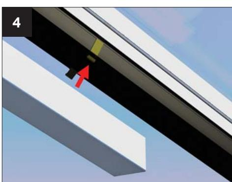
At the eaves push the ali undercladding on to the clips whilst ensuring they remain tight in the eaves.
