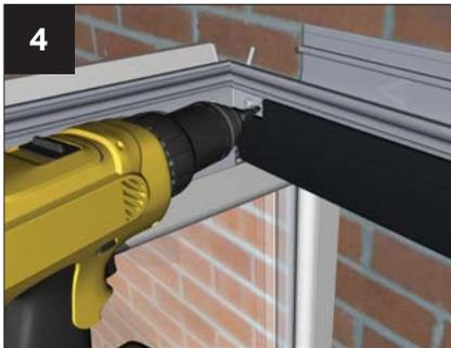
Either peel back or knife off a small amount of the insulation where the cleat is to be fixed. Drill a 4.5mm pilot hole and then fix the cleats with the two M5 12mm taptite screws provided. The protruding taptite screws will need trimming back prior to fixing the adaptor (alternatively, when its time to insert the adaptor, undue the taptites, drill a pilot hole through the adaptor and then re-screw the taptites and fully seal).
