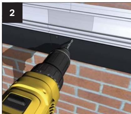
Drill through the top edge of the aluminium box gutter at 600mm centres. A fixing must be positioned within 50mm each side of the joint.
