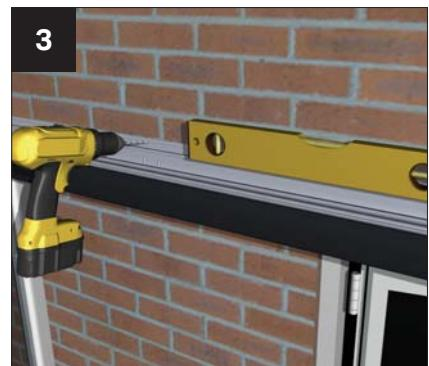
Whilst ensuring that its level, drill through the back edge of the aluminium at 600mm centres. Bolt to the house wall using masonry anchors that are suitable for the substrate.
