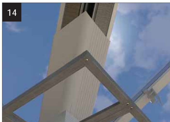
14 Measure and fit the standard valley undercladding NVU-V between the eaves and mark 'C'. Scribe to suit.
