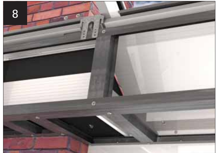
8 Fix the vertical frames in place using CHA006 (bag of 25) as per standard installation.
