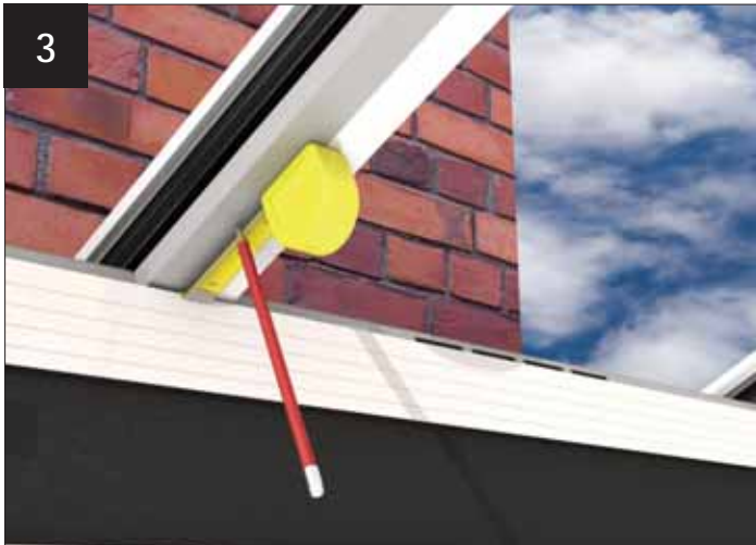
3 Using LHE---/2 as a datum, measure and mark the positions of the brackets in line with the dimensions given in the provided paperwork.
