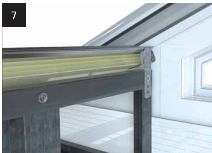
Fit the horizontal and vertical frames as shown in the main internal insulated pelmet installation guide. (pages 17 and 18).
