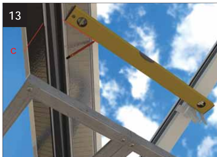
13 Using the bracket positions, level through and mark off the valley marked 'C'.
